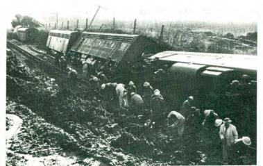
This is what happens when it rains, and rains, and rains. The roadbed turns into a mire and in unable to support the weight of a loaded train. Here, workmen make repairs
