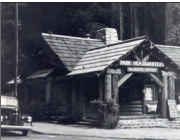
Big Basin ranger station.
