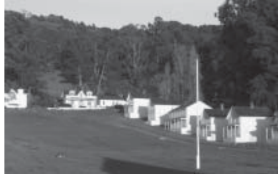
Civil war era buildings at Fort Reynolds >>
