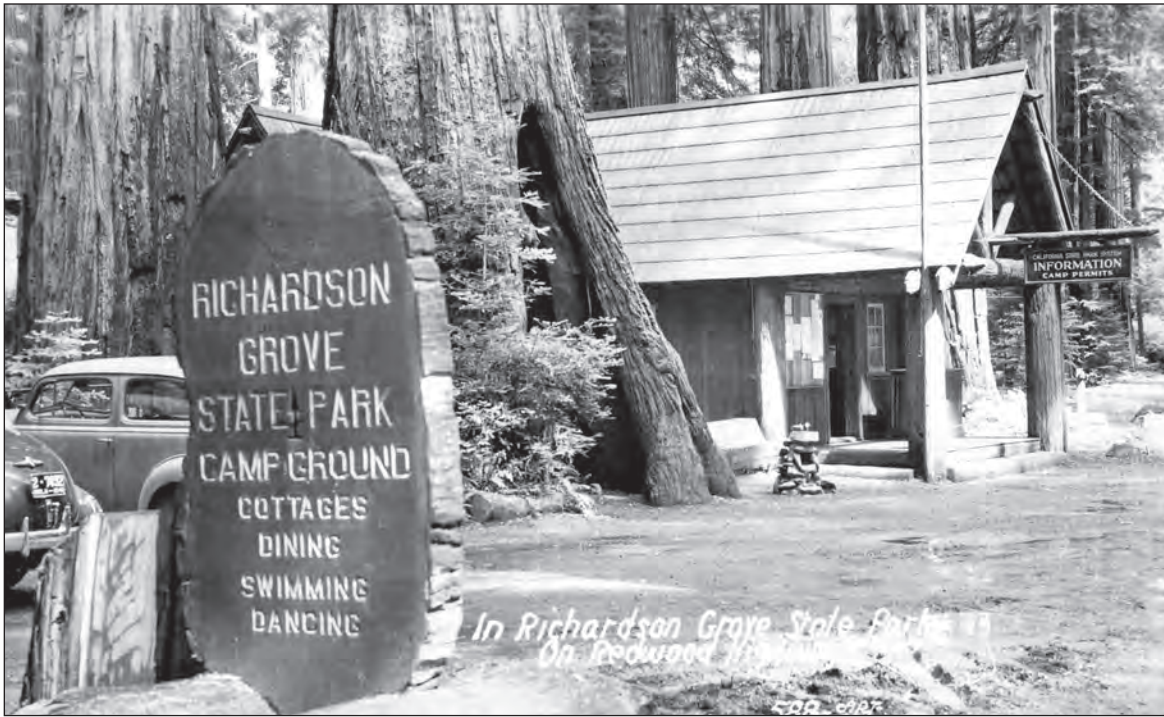
The Richardson Grove Ranger Station was right on the Redwood Highway, now U.S. 101.
