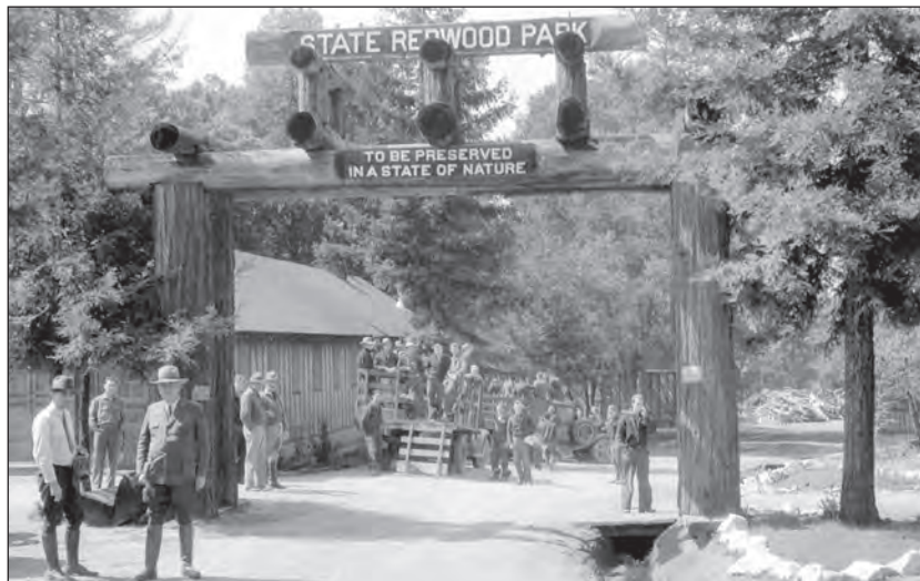
The CCC working at Big Basin. (Courtesy California State Parks.)
