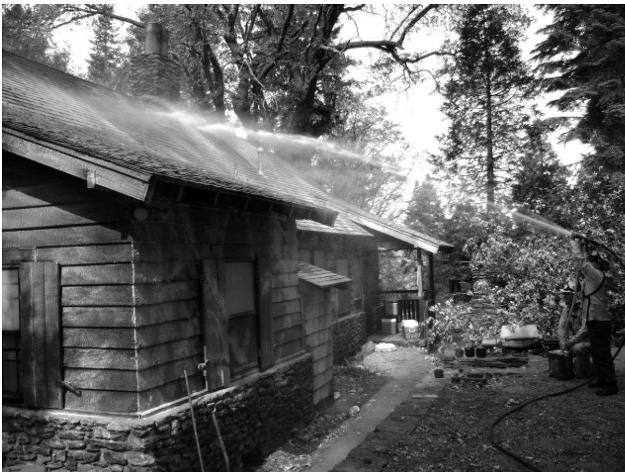
ThermaGel being sprayed onto the historic CCC-built park residence at Palomar Mountain SP
